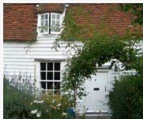
Typical details: weather-board, tiled gambrel roof, Bradwell-on-Sea
