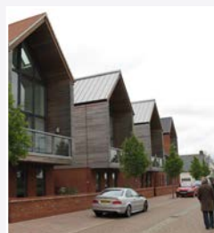
Roof overhangs providing protection to glazed facade
